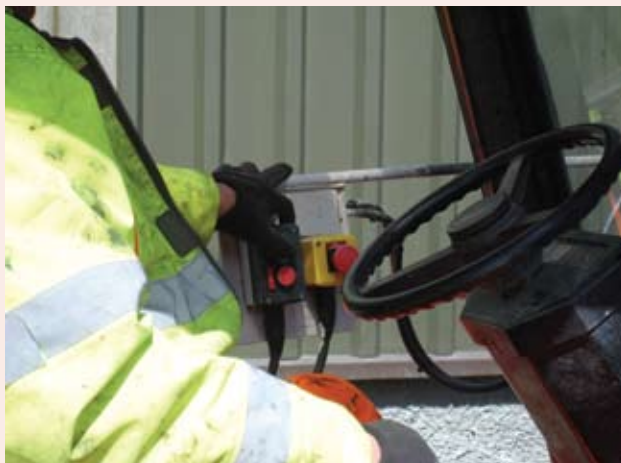
Above: New control pad
