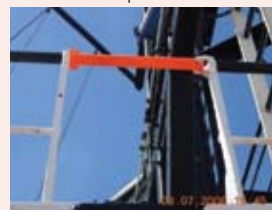
Previous fall protection
