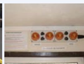
Shower alarm lights
