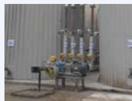
Bitumen lines - before
